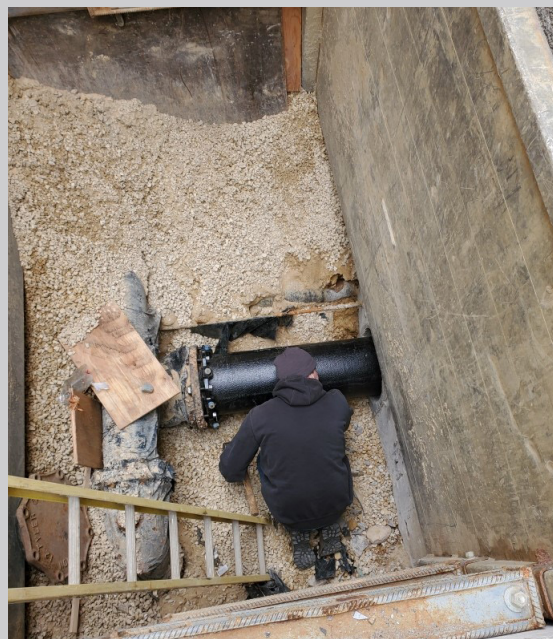
Physical Plant Steamfitters Kevin Corcoran (pictured) and Kevin Luginbuhl conduct an emergency repair of the 12-inch chilled water line where it enters the McArdle Building.
